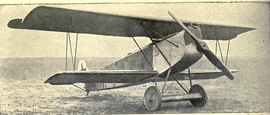
Fokker D 7. One of the most efficient single-seater fighting machines designed during the war.
